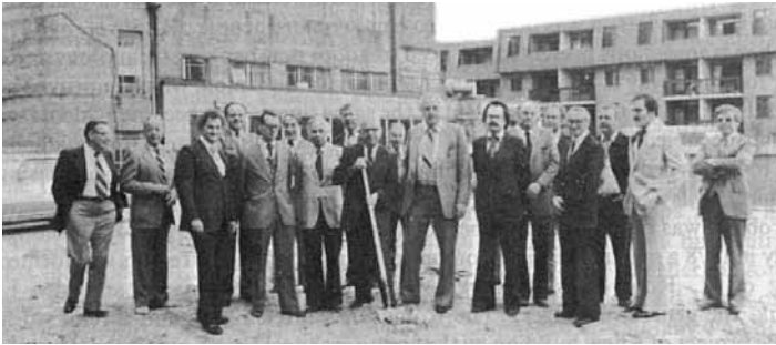
Former Chair of the UCU Board of Directors Wasyl Sytnyk (with shovel) breaks ground for the new UCU Head Office at 295 College St. Flanking him are architect Ihor Kotowych and Michael Rebryk the then serving Chair of the UCU Board, 1980.
